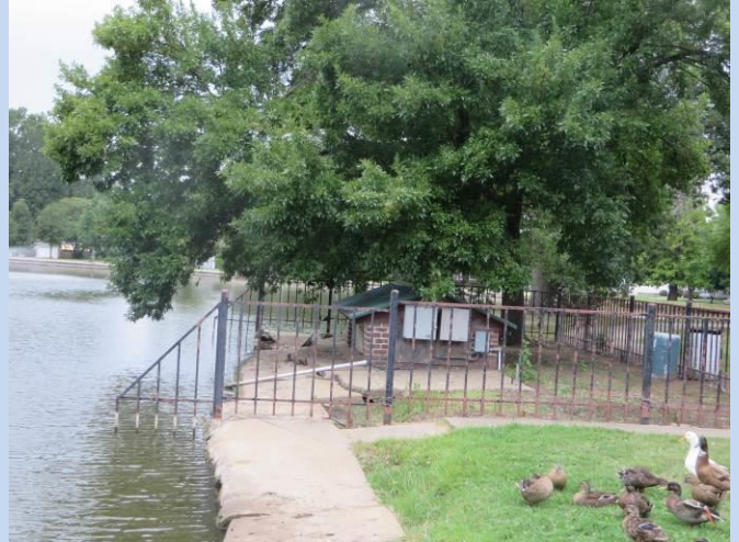
An additional benefit of the Lakeside Park project is the dilapidated duck house, broken concrete and unsightly fence will be removed. Hopefully problems created by too many ducks and geese will improve.
