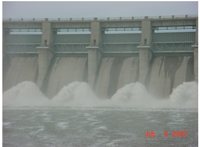
Toronto Reservoir stilling basin
